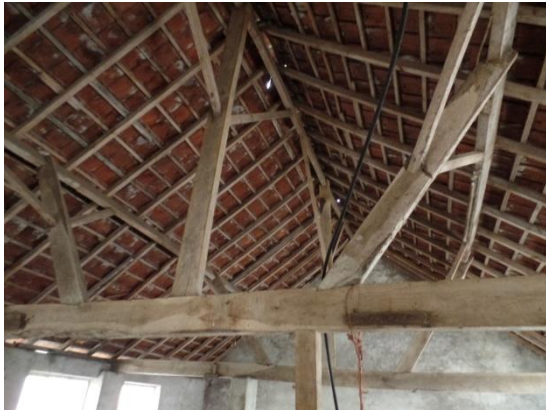
Fig.9 Dak zonder dakbeschoot
